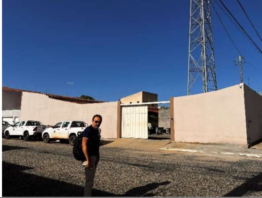
Office and Core Shed House 1 of the Lithium Ionic in Araçuaí-MG-Brazil – external view
